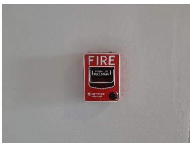
Fire Alarm Manual Station
